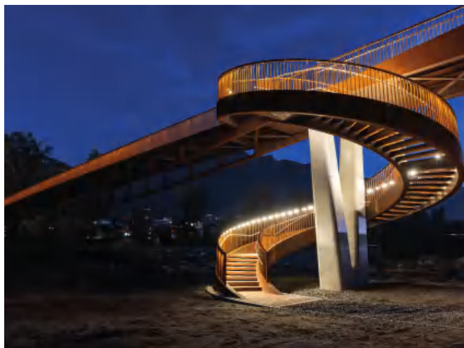
LaneLED WALL, Passerella Torretta Bellinzona
