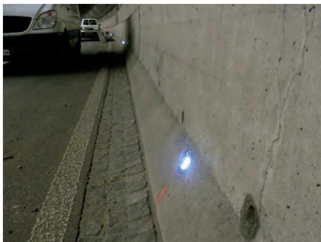
Tunnel Stephanshorn Saint-Gall
