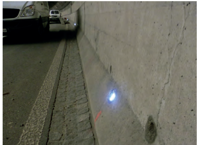
Tunnel Stephanshorn St. Gall
