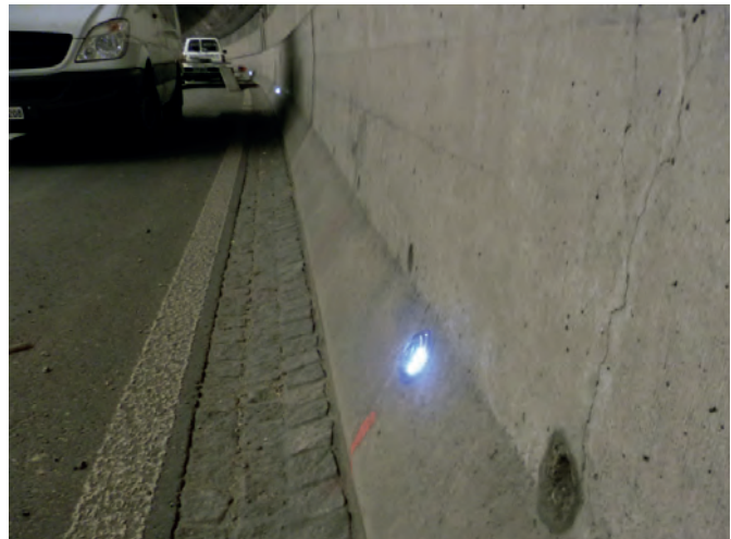
Tunnel Stephanshorn St. Gallen
