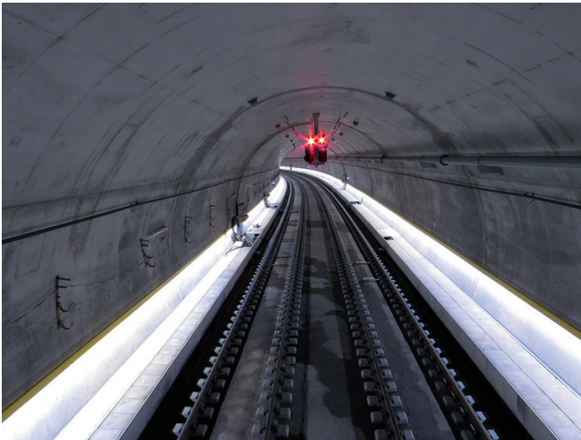
Overall view of SBB-cross city link Zurich
